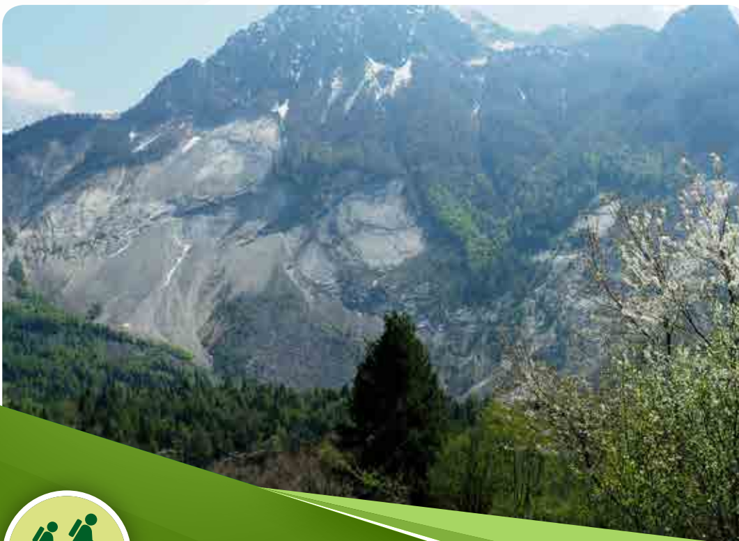
Monte Toc's landslide
